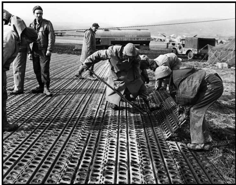
Runway Construction on Adak, 1942.
